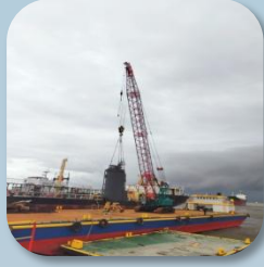
Barge Mount Crane
